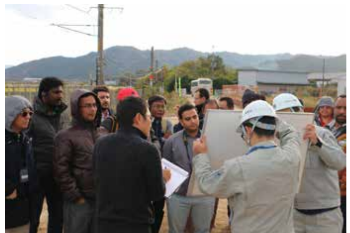
Trainees Learning about the Reconstruction Work of the 2014 Torrential Rain Damage in Tamba, Hyogo
