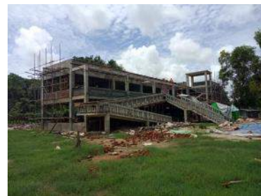
Completed the main framework construction of the school cum shelter
