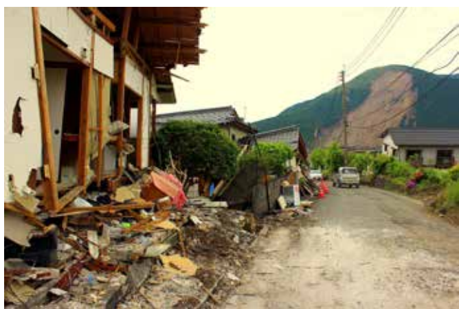
Damage in Minami-Aso. Many houses were collapsed at their first floor while landslides happened on a hillside
