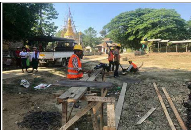
The Construction Site of the New School cum Shelter (March, 2018)
