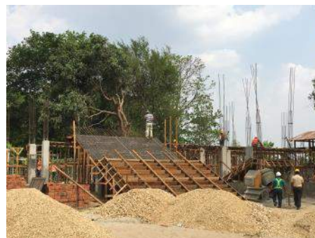
Construction site of the school cum shelter
