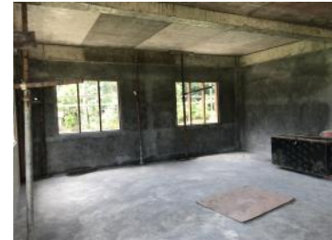
Class room of ongoing construction
