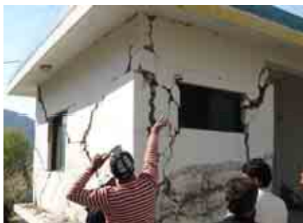
Photo 13 Field visit (damaged building)
