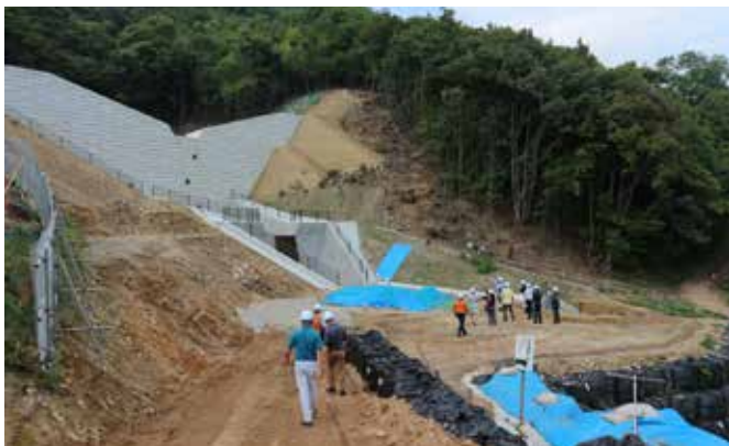
Visit of Sediment Controlling Dam at Hiroshima Sediment Disaster Affected Area
