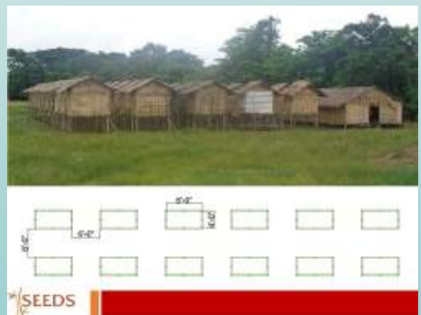
Temporary bamboo houses for construction workers
