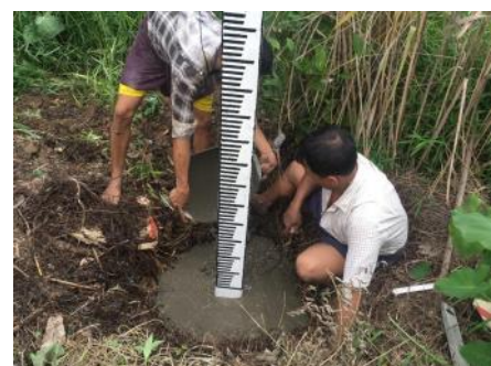
Installing water level measurement gauge
