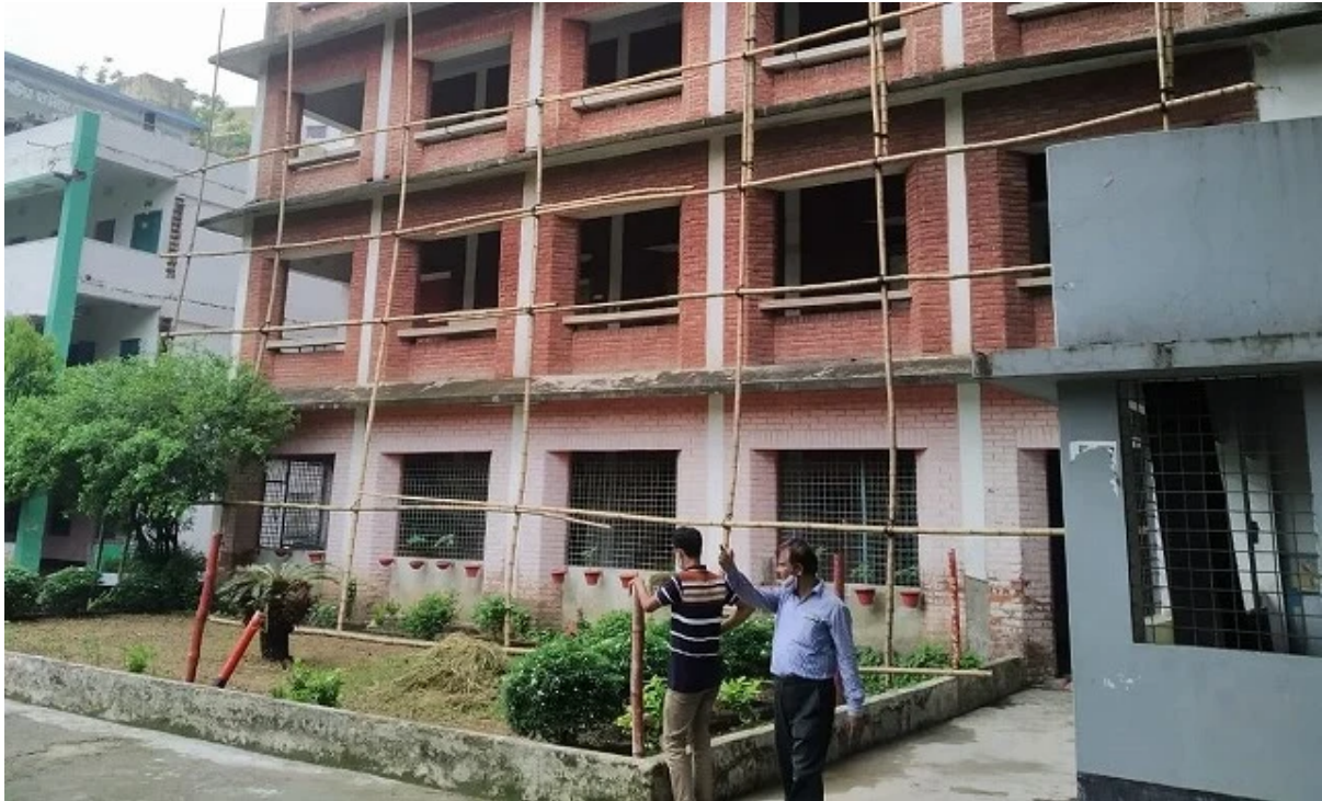
Preparation of rainwater harvesting system installation at Lalmatia Housing Society School and College [Bangladesh]
